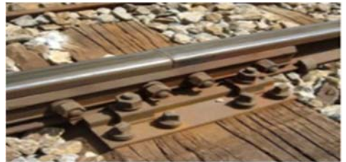
Fig. 5.1.2.2(a) One meter Long Fish plates
